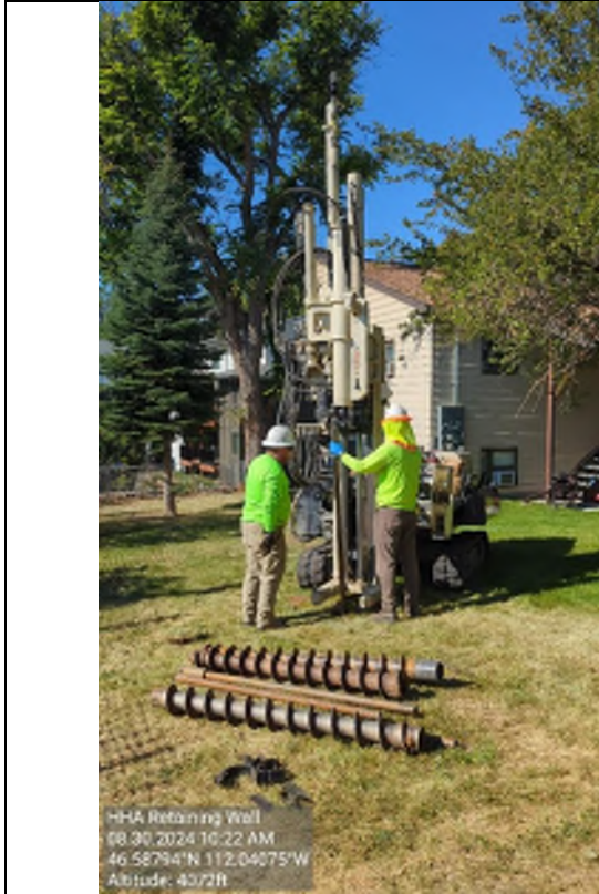
Picture # 1: Drill Rig Location
